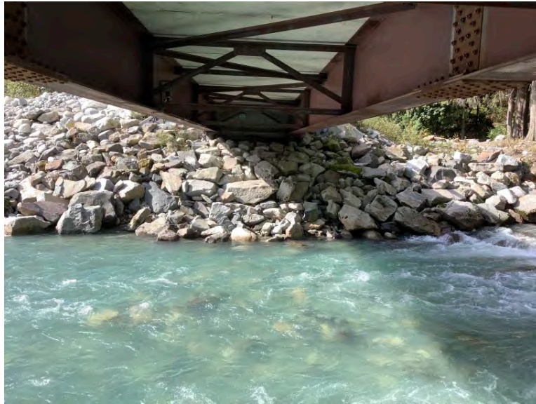
Right Bank Abutment when facing downstream
