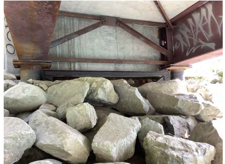
Left Bank Abutment when facing downstream
