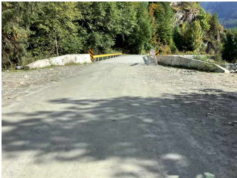
Approach from Right Bank when facing downstream
