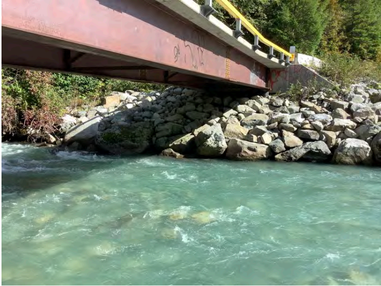
Left Bank Abutment when facing downstream
